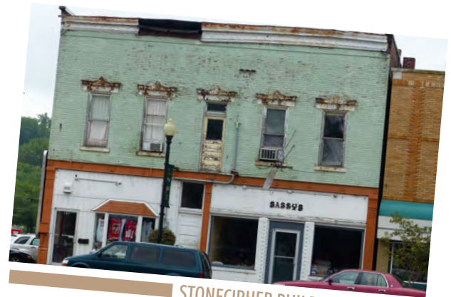
STONECIPHER BUILDING CONDITION
