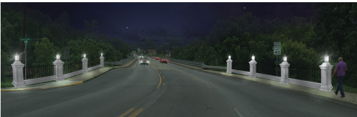
Night view of gateway lighting on Indian Creek Bridge on Capitol Avenue
