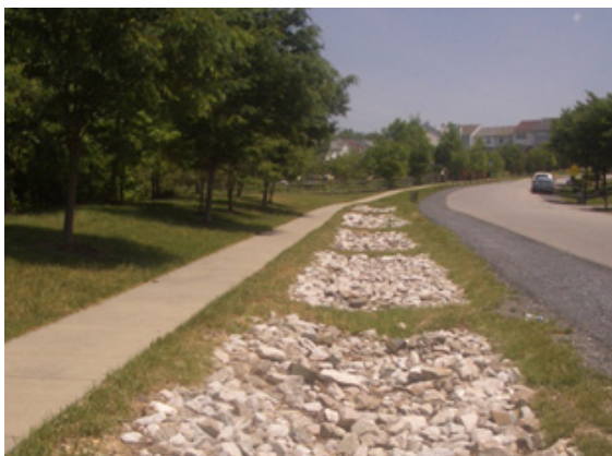
Infiltration trench, sustainablestormwater.org
